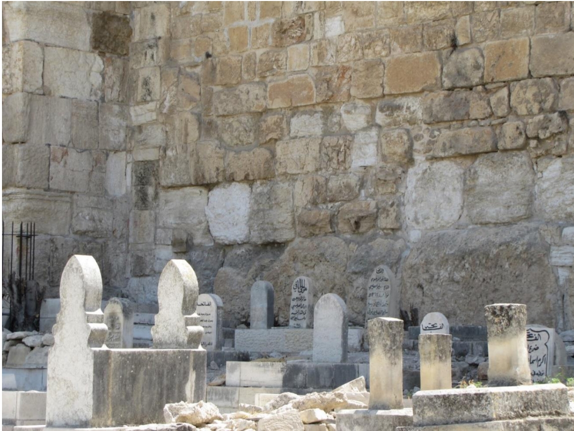
View of stones (large bottom row) from the Corner Tower remaining from Babylonian destruction and used by Nehemiah in Corner Tower of 444 BC
