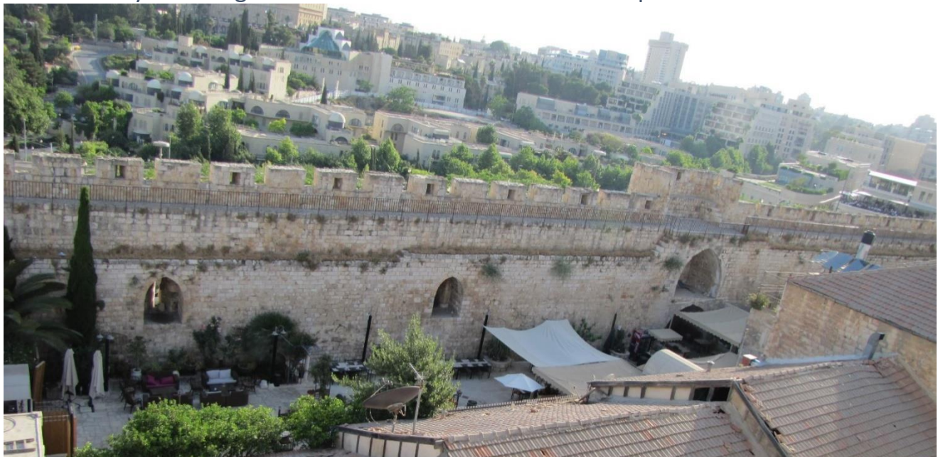
Space to walk on the inside of the west walls of Jerusalem on the west side of the Western Hill. The Hinnom Valley is on the other side of these walls. Built 1537-1541.
